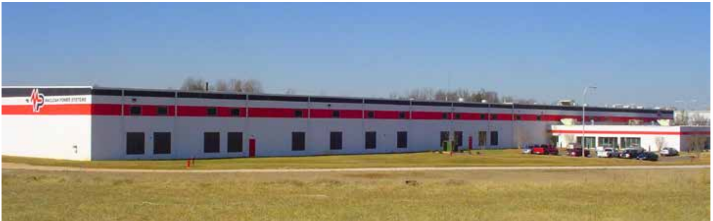
MacLean Power Systems — York, South Carolina
