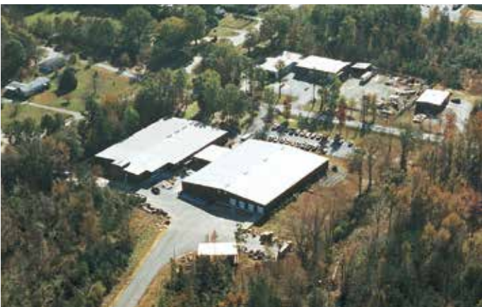
MacLean Power Systems — Newberry, South Carolina
